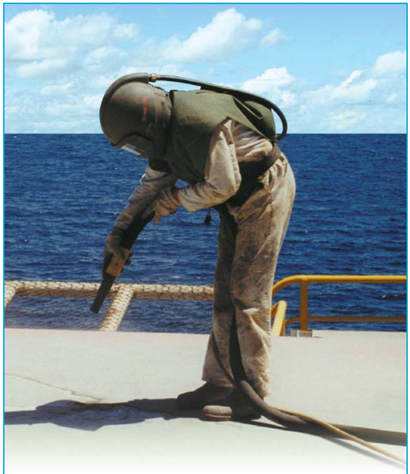
Blasting with Blast-One SpeedBlast™ is faster, cleaner and lot more neighborly.
