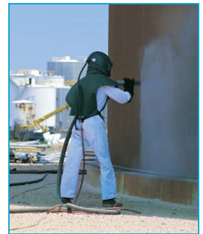
Blasting with Blast-One SpeedBlast™ is clean and fast!
