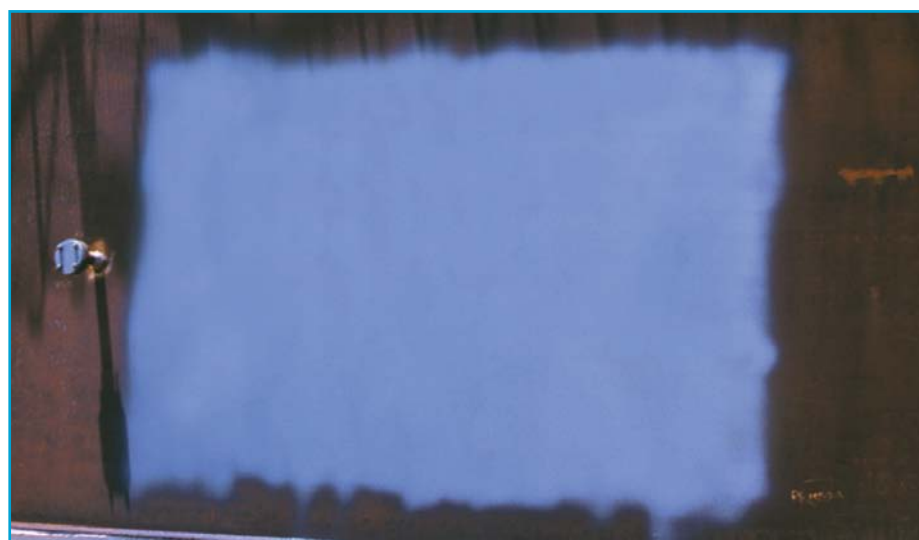
15 minutes blasting with Blast-One SpeedBlast™: 60ft 2 blasted – 125 lbs used. Amazing!
